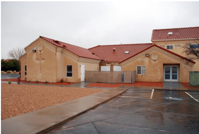
Back of Fellowship Hall and New Entry
